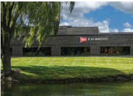
ITW Orbital Cutting & Welding U.S. Headquarters
